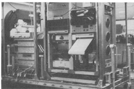
Fig. 52. Clock box and timing electronics being mounted in framework.
